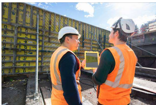
Site manager Christian Hänni (left) and BIM manager Stijepan Ljubicic (right) from STRABAG AG check the formwork construction on the 3D model.
